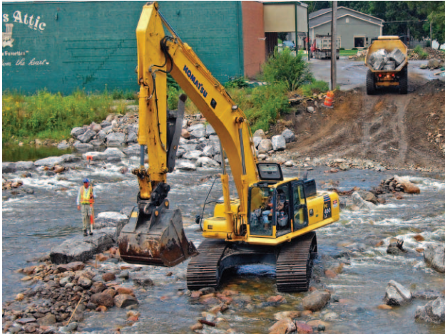
Construction of Chesaning weirs
