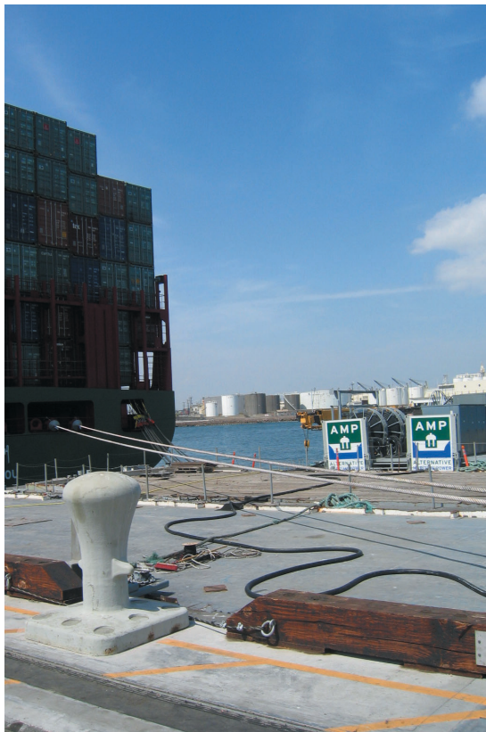
Long cables connect a large container ship to shoreside power.
