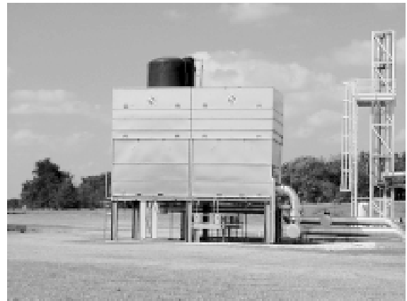
Diesel generator located at the Eagle Mountain International Church outside Fort Worth
