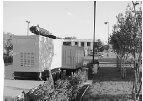
Two diesel generators in close proximity to a children's playground in Richardson
