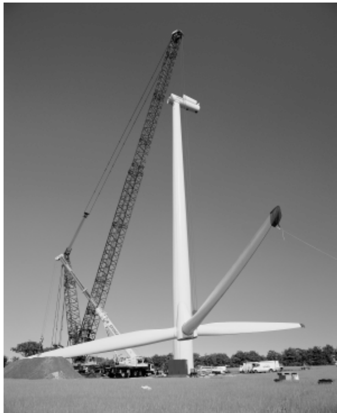
Turbine construction. Photo © BONUS Energy A/S.
