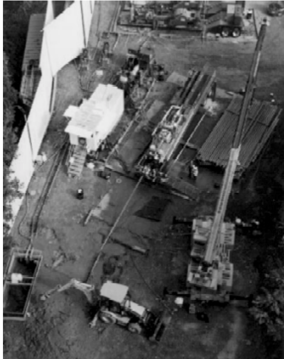
Aerial overview of a typical directional drilling site. 17
