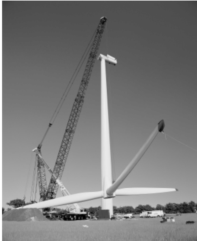
Turbine construction. Photo © BONUS Energy A/S.
