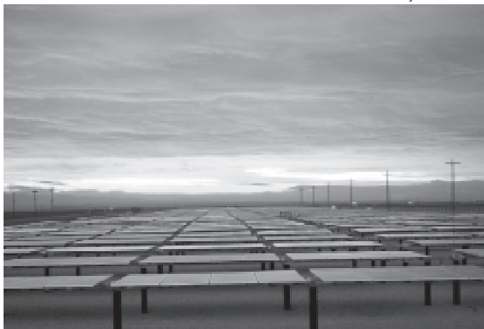
A utility scale installation of solar panels.
