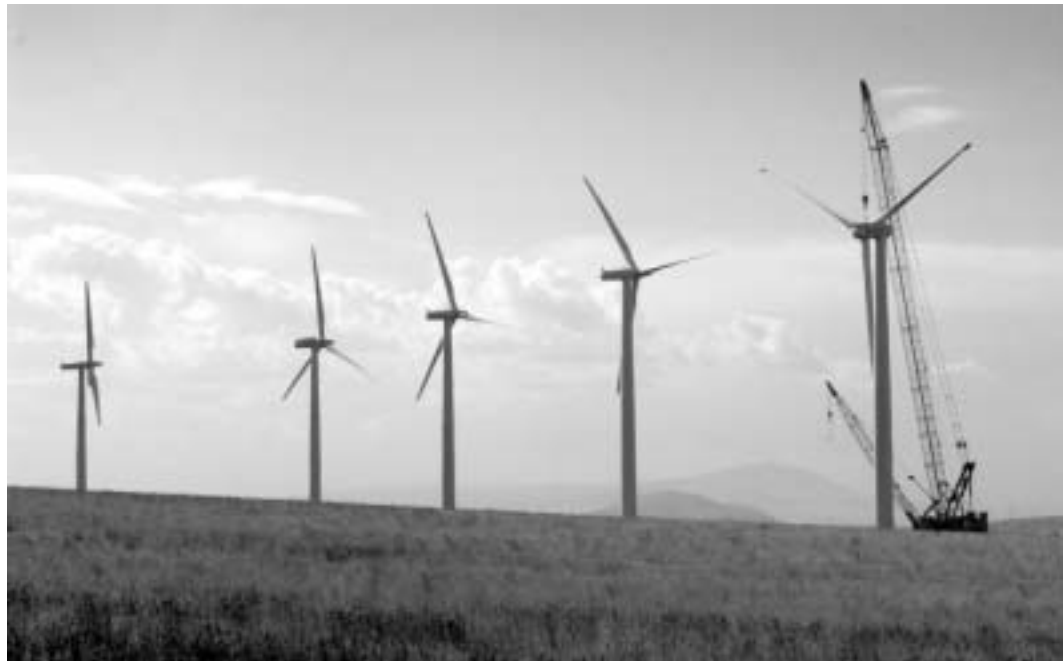
Wind turbines at Nine Canyon
