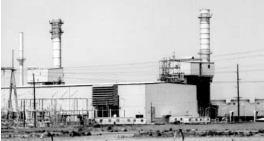
A natural gas power plant.
