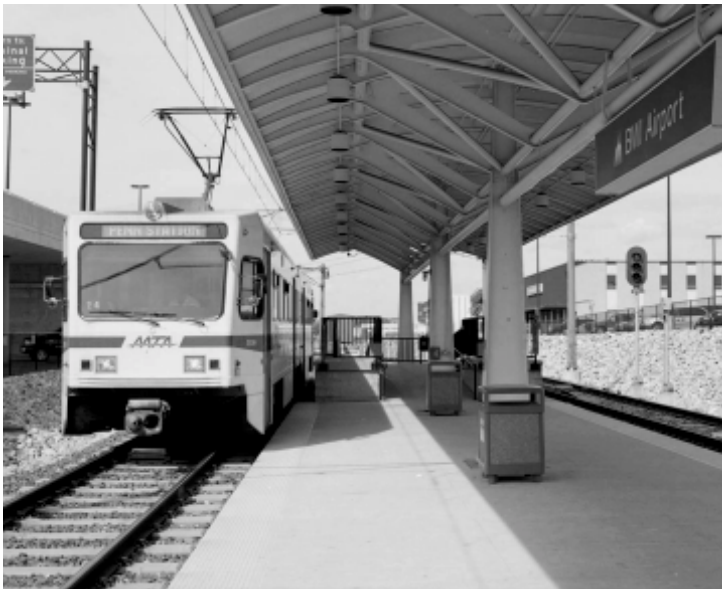
Light Rail stop at Baltimore-Washington International Airport
