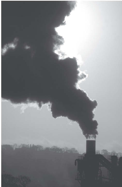
Florida's 13 coal-fired power plants are the largest source of mercury emissions in the state.
