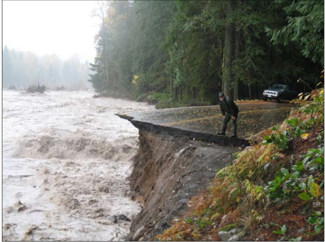
November 6 and 7, 2006. After a massive rainstorm which dropped 18 inches of rain on Mt. Rainier National Park in Washington, the Nisqually River raged in flood. The rushing water destroyed more than 200 yards of the main park road and wiped out Sunshine Point Campground.
