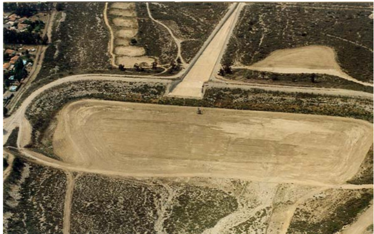
Fig. 8. Deer Creek Debris basin and concrete spillway. Note residential development at left. Two dry channels of Deer Creek are visible at the bottom of the photo. At top, pond-shaped catchment basins flanking the spillway store water in wet years for recharge to underground aquifers.
