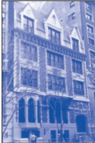
The Makor building, on West 67th Street in New York City.
